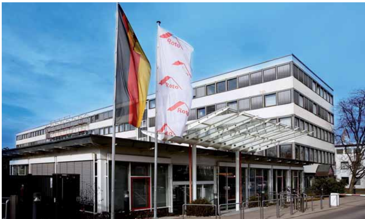
Entrance area of the Leinfelden-Echterdingen production plant
