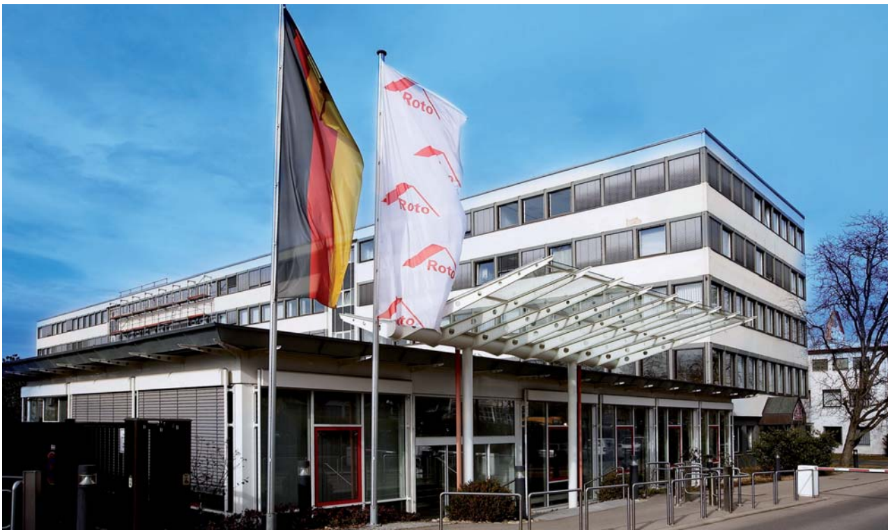
Entrance area of the Leinfelden-Echterdingen production plant.
